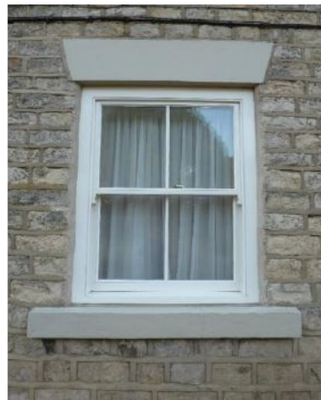
Modern sash window
