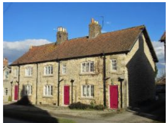
Cottages in High Street
