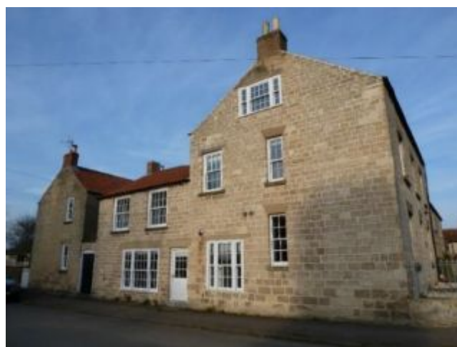
Lime pointing at Prospect House
