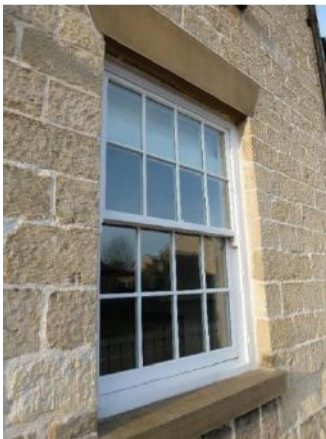
Modern sash window
